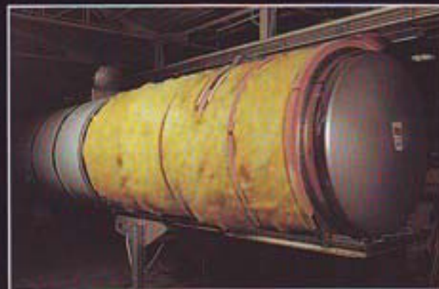
6" Fiberglass Insulation, Compressed To 5"
